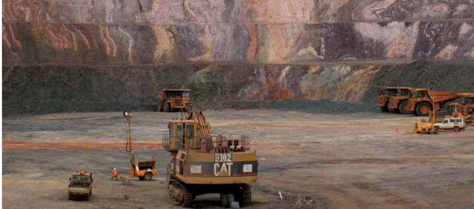
Figure 3: Geita Mine Pit being excavated
